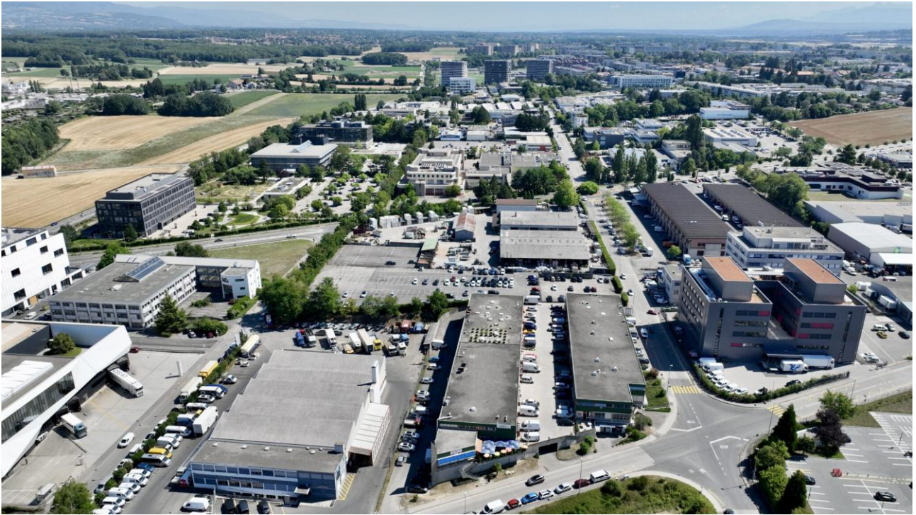
Aerial view of the Meyrin-Satigny-Vernier industrial zone (ZIMEYSAVER) | 2022: thousands of square metres of dark flat roofs, exposed to full sun, absorbing heat instead of reflecting it. ©FTI – Olivier Riethauser
