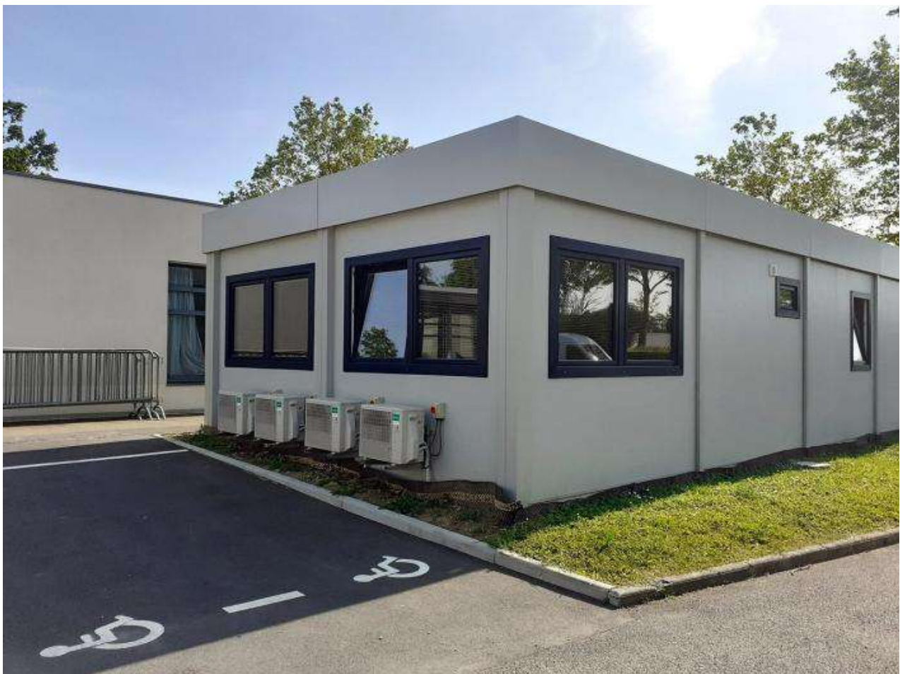
Temporary offices, administrative pavilions, modular classrooms: with low inertia, these structures overheat fast. Treating the envelope is the most effective lever to make them liveable, summer and winter alike.
