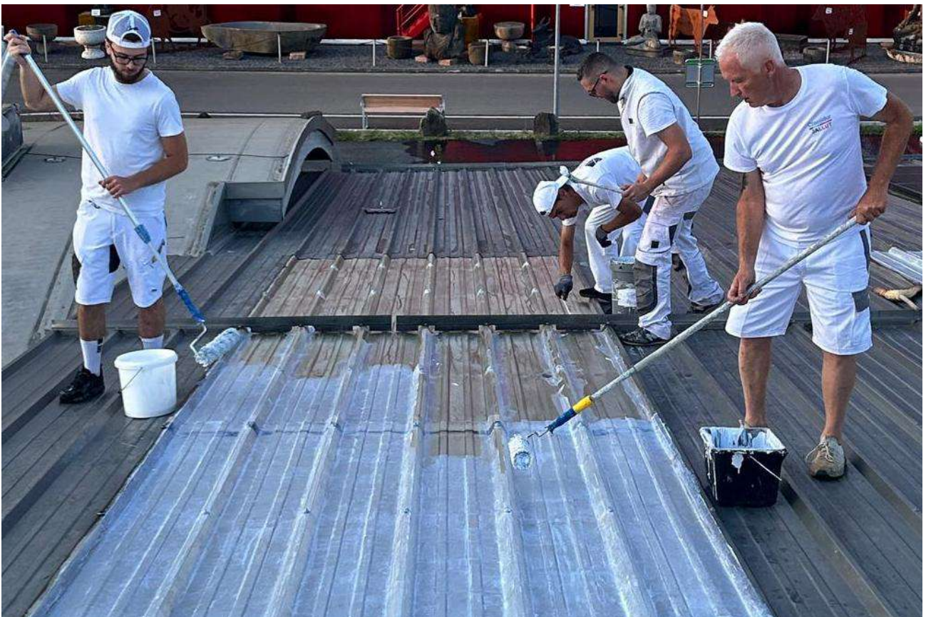
A translucent lacquer on the supports: it reflects solar energy while letting visible light through. Even, controlled shading, where the chalk remained approximate and messy.
